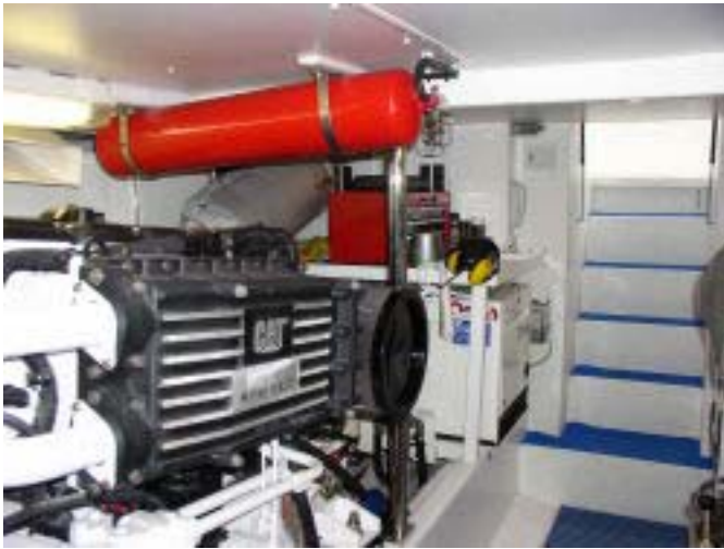
Engine Room to Starboard
