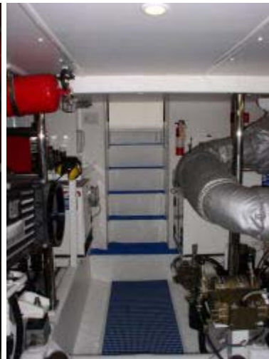
Engine Room Access
